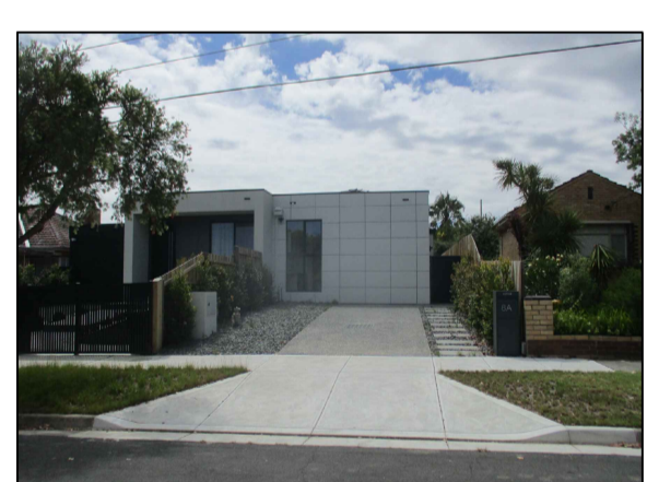
Photo # 10: No. 8A Example Street
